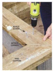
Add capping and finish Square cut and mitre the capping, apply construction adhesive to the ends and secure to the sleepers with 75mm x 14g galvanised bugle screws then use a router with a roundover bit to remove splinters and trim the edges. Apply two coats of decking stain.
